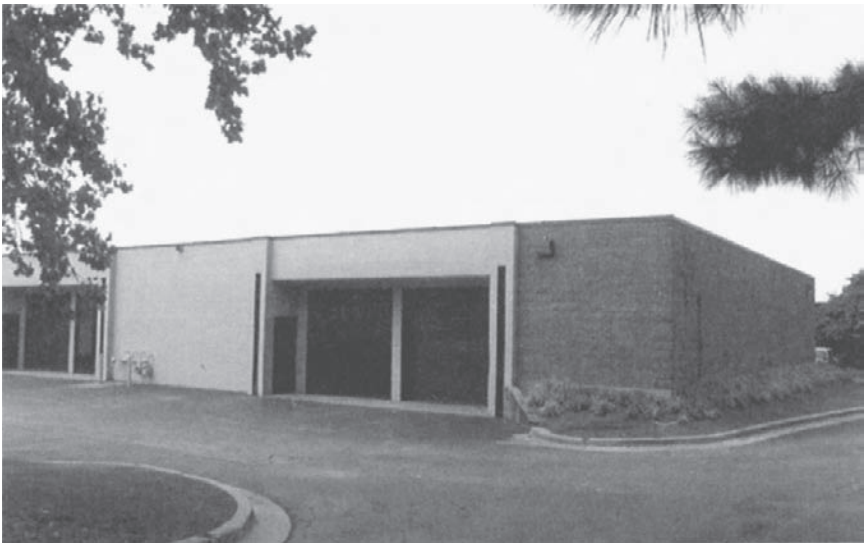
Figure 7.4. It is critical that the archaeology laboratory be accessible to field vehicles. Office parks are designed for this. In this picture, the “garage door” is the right-hand opening. The equal-sized area to the left is the tinted glass for the firm’s laboratory, shown in figure 7.1. (Photo courtesy of Paul Brockington and Brockington and Associates, Inc.)
